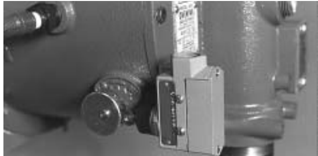
Low Fire Start Switch shown
